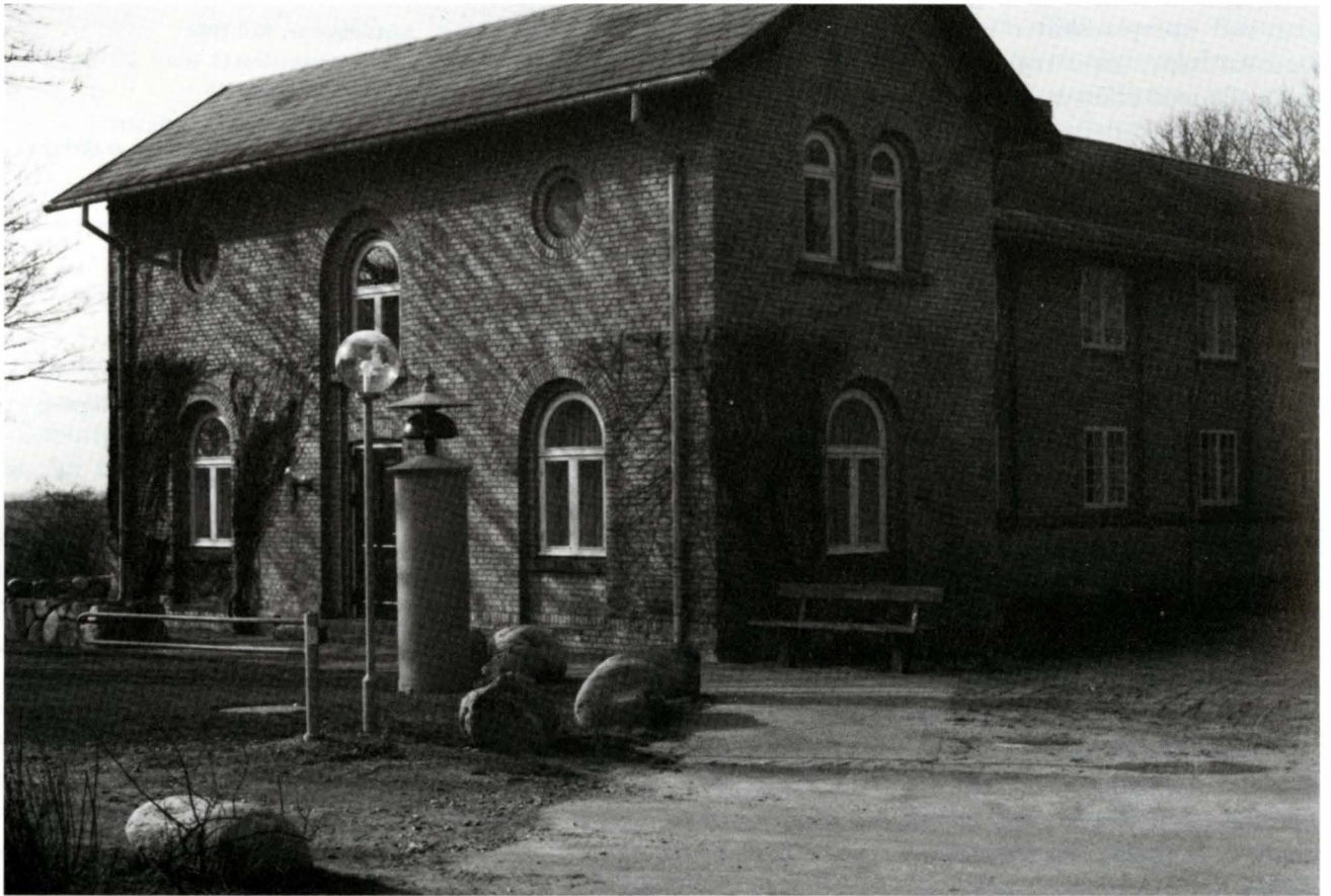
Den gamle remise. Knudshoved. Kursuscenter.
