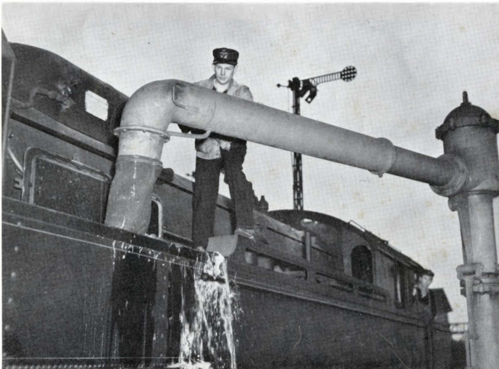
Lokomotivet vandforsynnes (vore store lokomotiver tager ca. 25 tons vand ad gangen).
